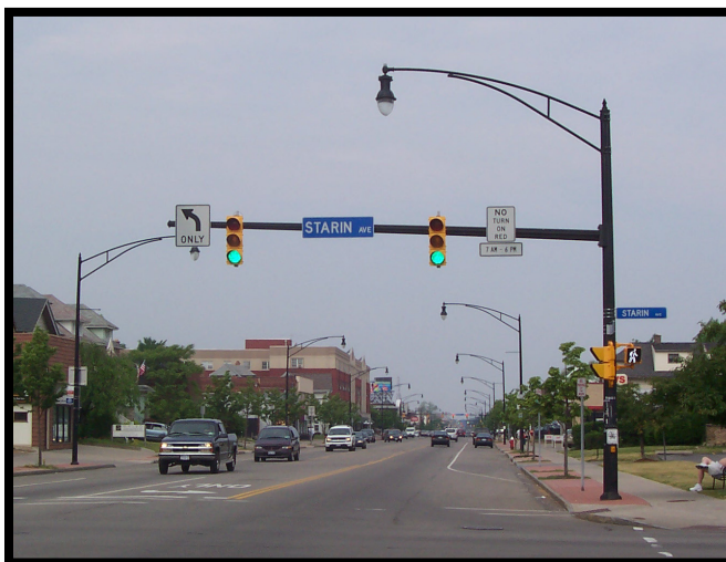
New streetlights and traffic signal mast arms, Hertel Avenue, Buffalo, NY.
